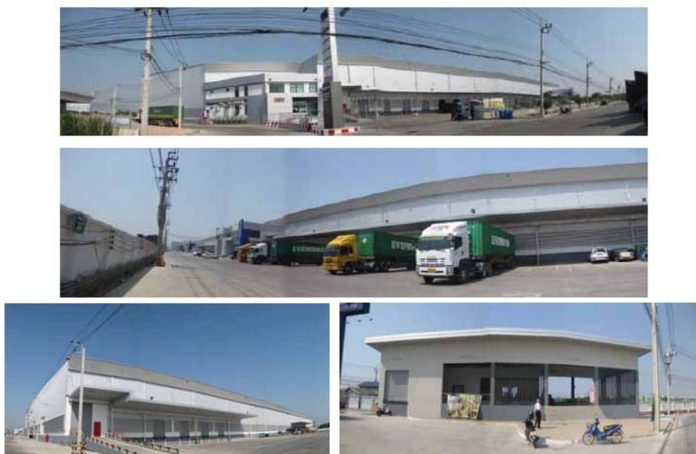
Picture 2 : Warehouse buildings and office of WHA Ladkrabang
